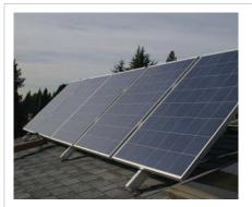
These solar photovoltaic panels are installed on a house in Burnaby. When the panels produce more electricity than is needed by the house, the excess is exported to BC Hydro through net metering. Source: Vancouver Renewable Energy Co-op
