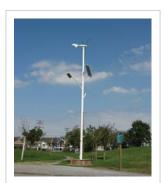
The City of Richmond is testing a new type of lighting system, generating both wind and solar energy, and storing the electricity to a battery to power the street light at night. Source: City of Richmond a building, is a way to avoid potential technical problems associated with building mountings.
