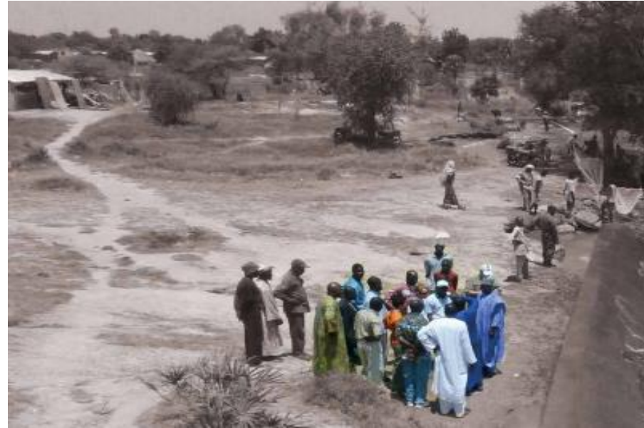
Assessing a dike at risk of collapsing in Cameroon due to heavy rainfall and flooding in August 2012.
