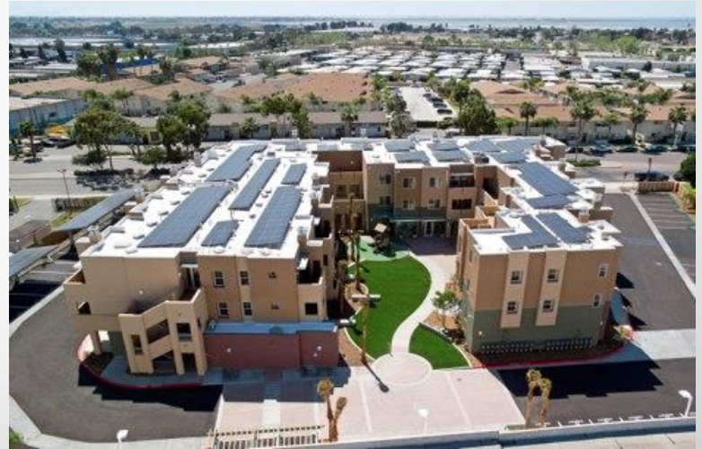
Los Vecinos, San Diego's 1 st LEED-certified Platinum, 100% solar-powered affordable housing.
